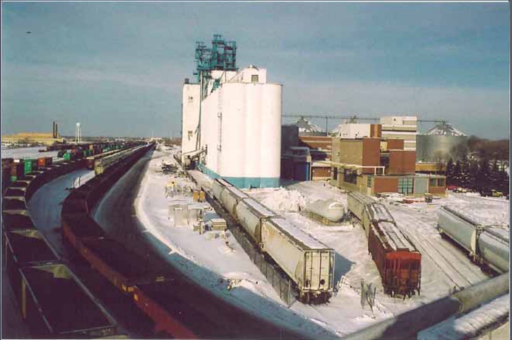
General Mills – Fridley Mill & Elevator
