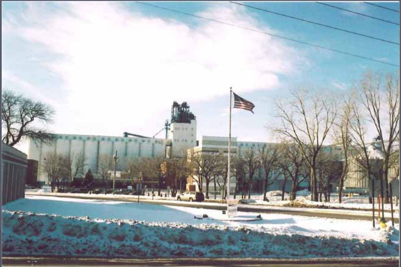
General Mills – Fridley Mill & Elevator
