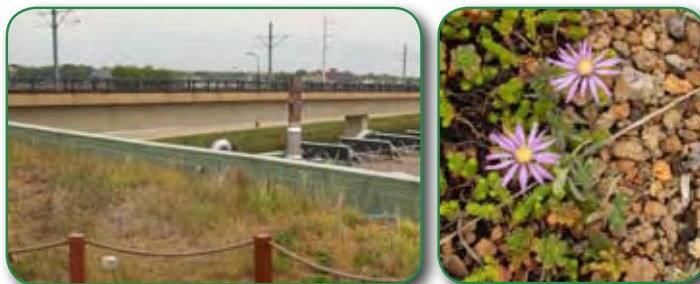
PEEC green roof with the Hiawatha LRT Trail in the background., roof detail on left.
