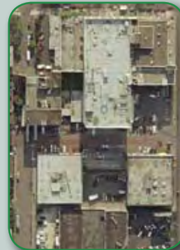
Seattle: typical flat roof
