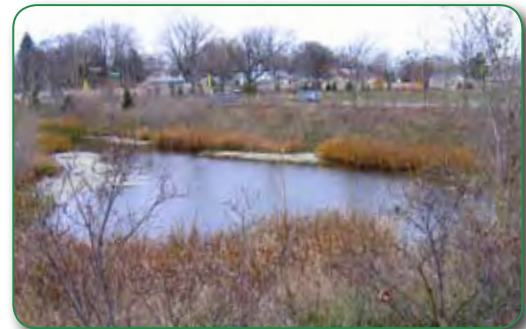
Ponding for regional/state highway constructed by Mn DOT.
