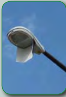
Full cut-off fixtures help control light pollution. Source: www.astronomybuff.com .
