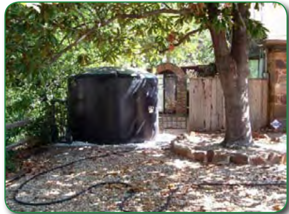
Rainwater harvesting systems collect and store rainwater for non-potable uses such as irrigation or toilet flushing.
