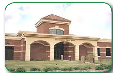
The new ultrafiltration plant in Columbia Heights is part of the City's water treatment system.
