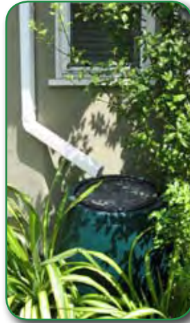
Rain barrels reduce runoff and can be used for home watering. Source: picasaweb.google.com/buildgreeninfrastructure
