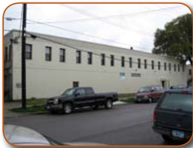
Industrial building in the Corridor
