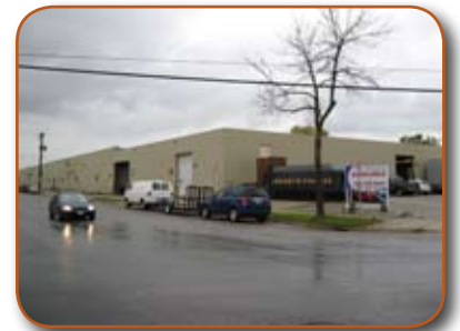
Industrial building in the Corridor
