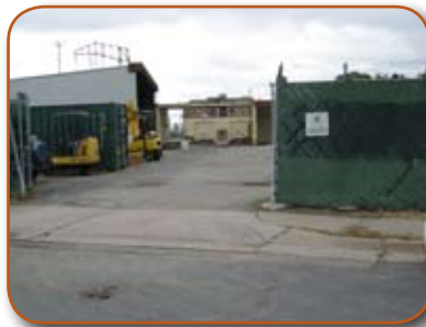
Industrial building in the Corridor
