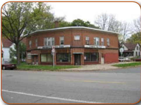
Retail space in corridor
