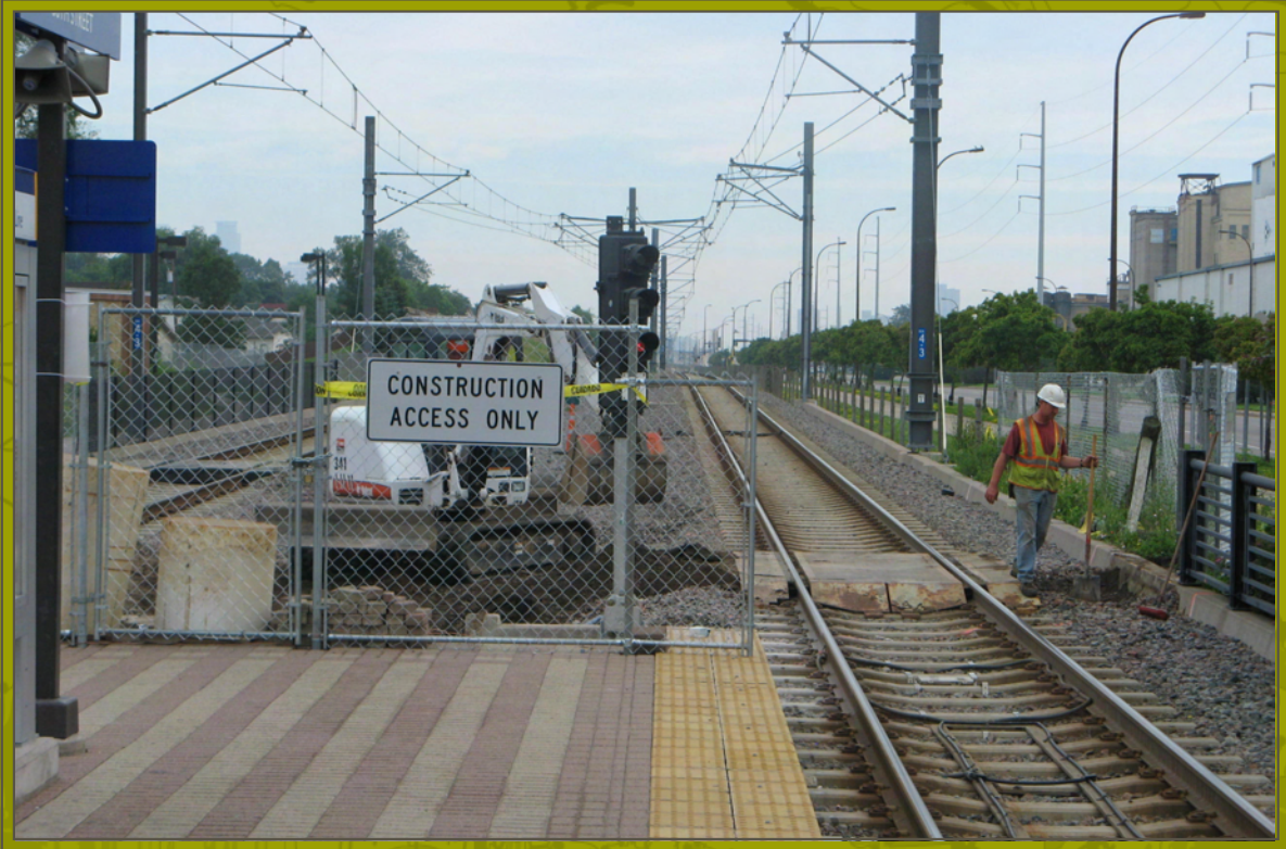
Improving the 38th Street Station platform
