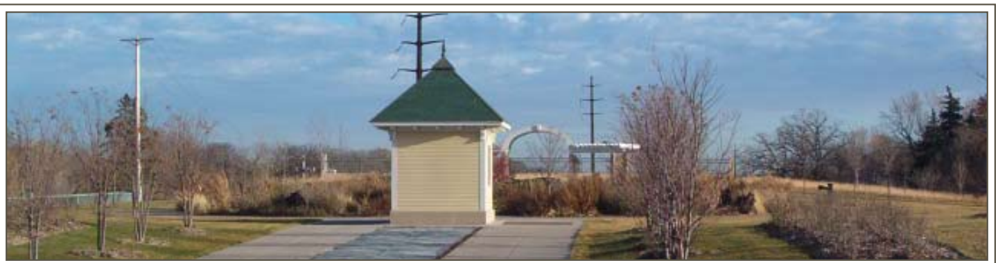
Longfellow Gardens is a new park built over Hiawatha Avenue/MN 55 when the highway was reconstructed.
